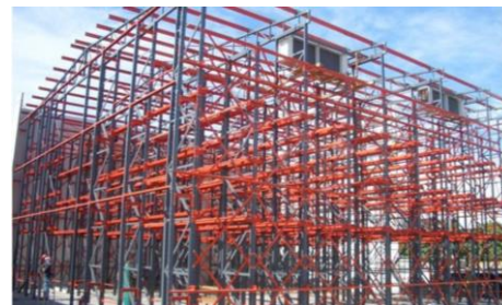
RACK SUPPORTED BUILDINGS
